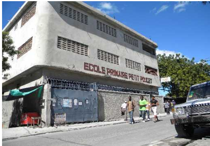
The front side of the collapsed school building.
