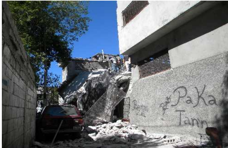
The rear side of the building that totally collapsed, seen from the side alley.
