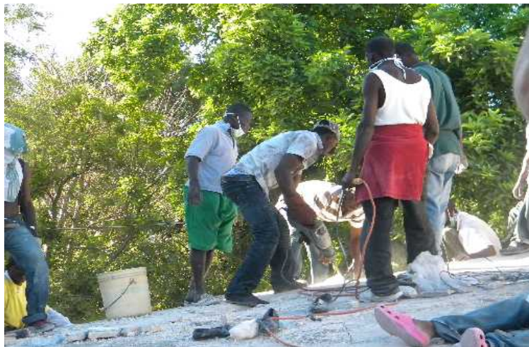
When an electric generator and power tools arrived, these Haitian men found “new strength.” PTL
